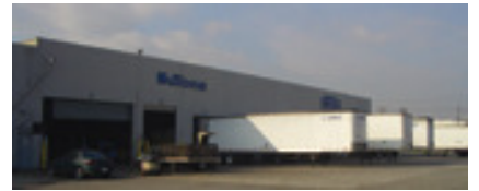
Rexford Industrial has purchased a 191,466-square-foot industrial building in Vernon, Calif., for $14.5 million.
