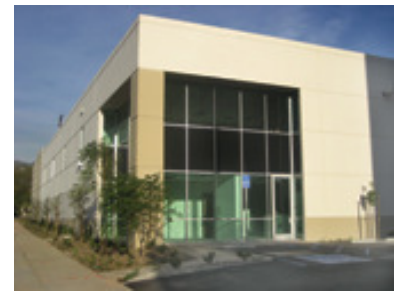
Rexford Industrial LLC has completed the redevelopment of a 113,477-square-foot industrial project located in Sylmar, Calif.
